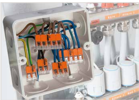
Wiring fine-stranded conductors in a junction box.
