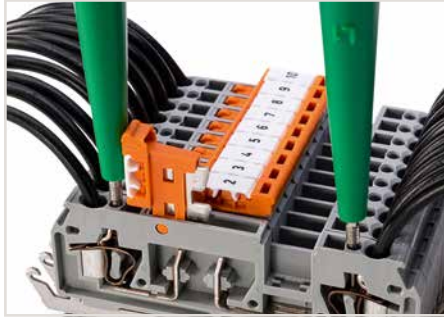
Testing with voltage tester.
