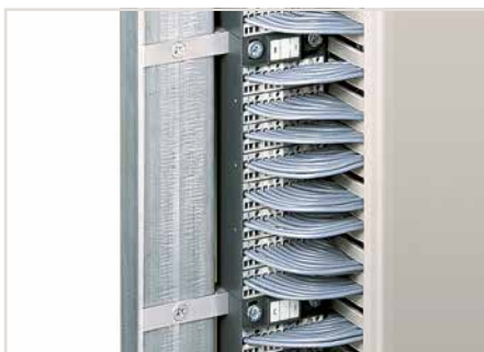
Installation example: Matrix patchboards in a frame
