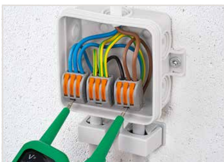
Testing the wired connectors.
