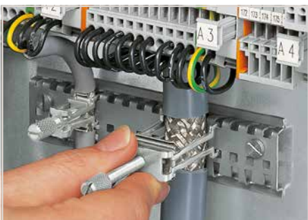
Fitting an additional clamping saddle.
