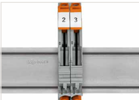
Preparing shorting path for the current transformer circuits.
