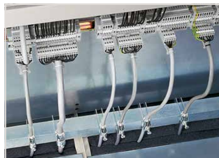
Cable entry in the base of the switch cabinet, with separate strain relief, movable IP54 bottom plates sealed with sponge rubber (e.g., by Rittal)
